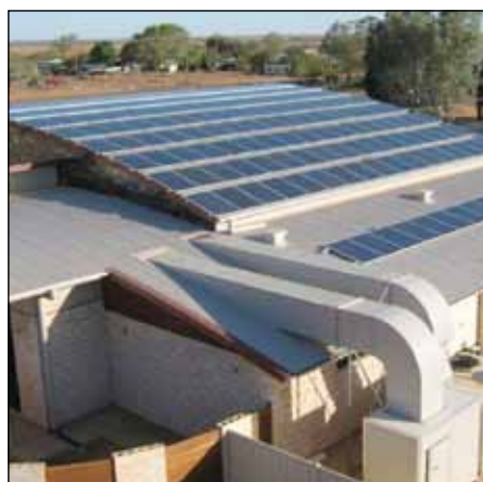
Windorah Cultural Centre roof fitted out with an Ingenero solar system.
