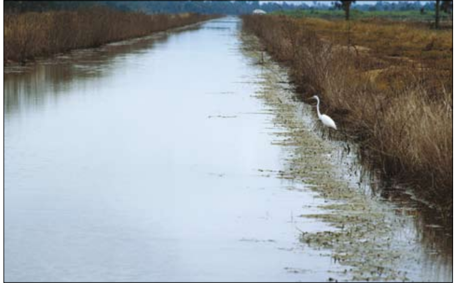
An irrigation supply channel near Clare in the Burdekin Valley, Queensland. An enzyme developed by CSIRO shows promise at removing the herbicide atrazine from irrigation run-off.
